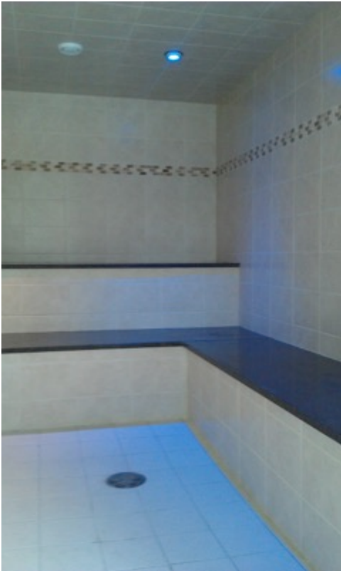
Large format wall tiles with granite seat tops
